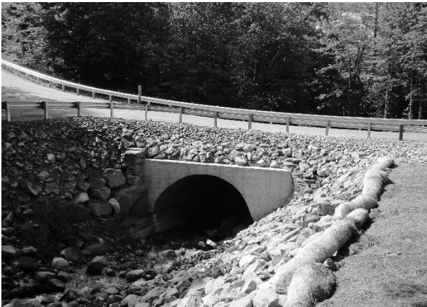
Basin Bridge after reconstruction by NH DOT
